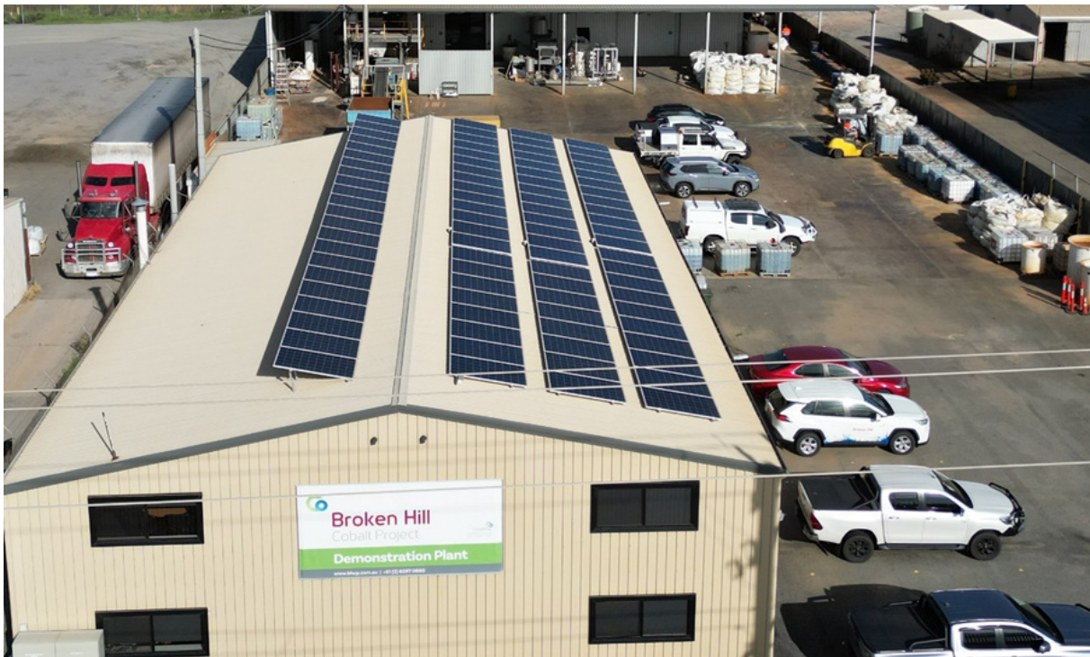
Figure 2 - Aerial view of the Broken Hill Technology Centre.
