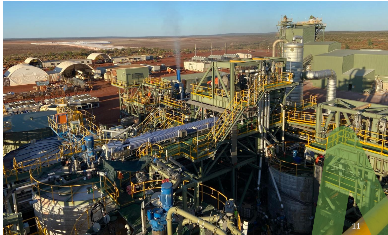
Beyondie SOP Plant in operation during Reward due diligence site visit in August 2023.
