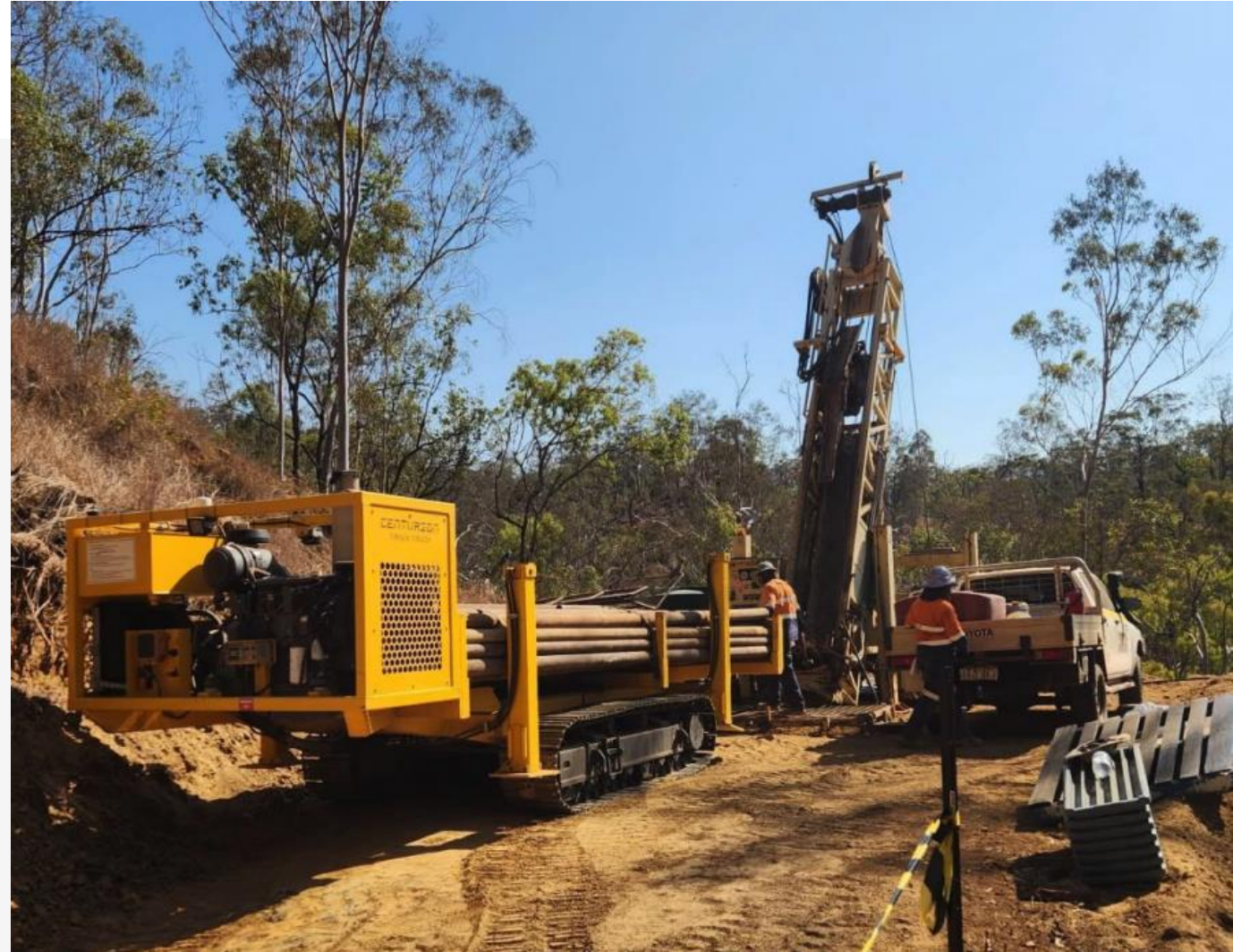
Drilling on site at Specimen Hill, QLD, October 2025
