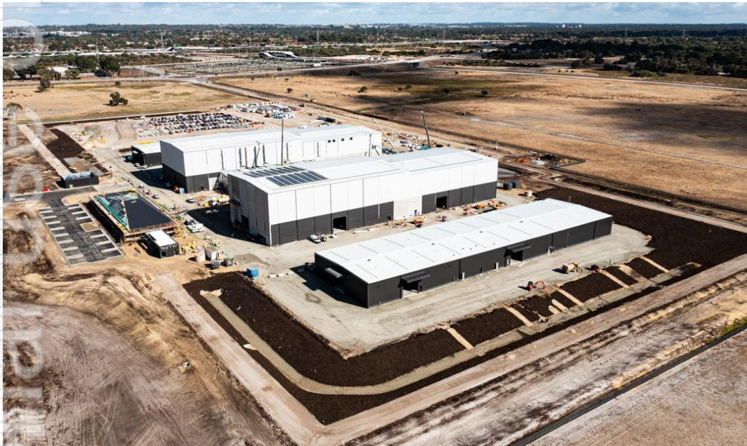
Malaga Film Studios under construction 2024
