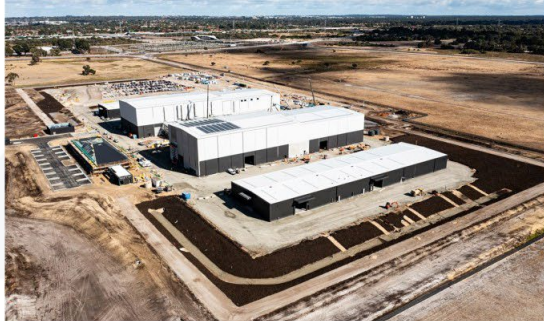
Malaga Film Studios under construction 2024 * Image courtesy of Built Pty Ltd
