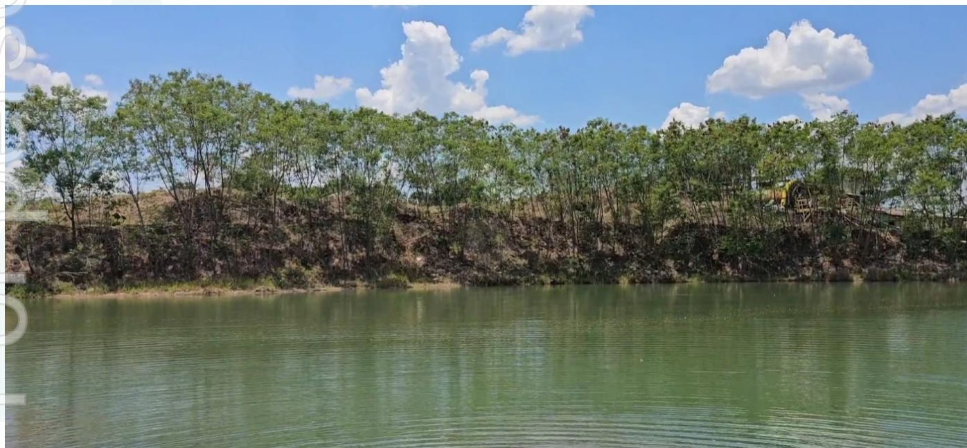
Figure 13: Tailings material (approximately 10m high), (left), relative to 30tph processing plant (right).
