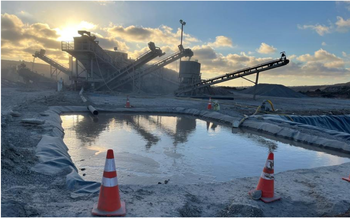
Image 3: Water recycling pools for plant operations
