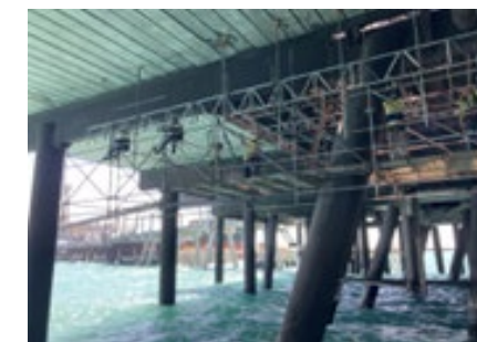
Scaffolding in place for Pile Wrapping Project
