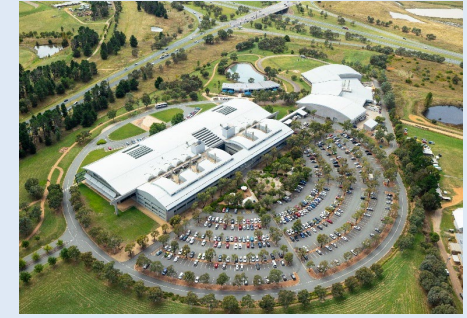
Geoscience Australia Facility, Canberra (CLW, CQE & DIF4)
