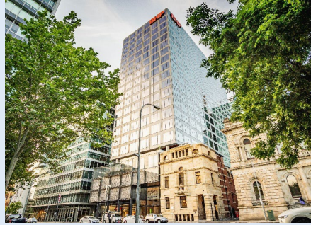
GPO Tower, 2-10 Franklin Street, Adelaide (CPOF & CHWPT)
