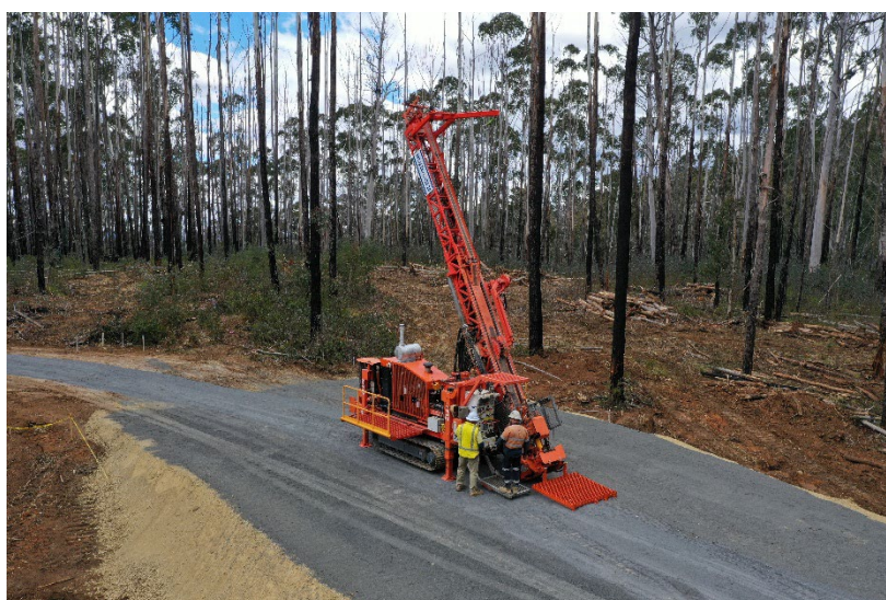
Figure 1: Eagle Drilling NQ Pty Ltd commence drilling at the Pilot Project
