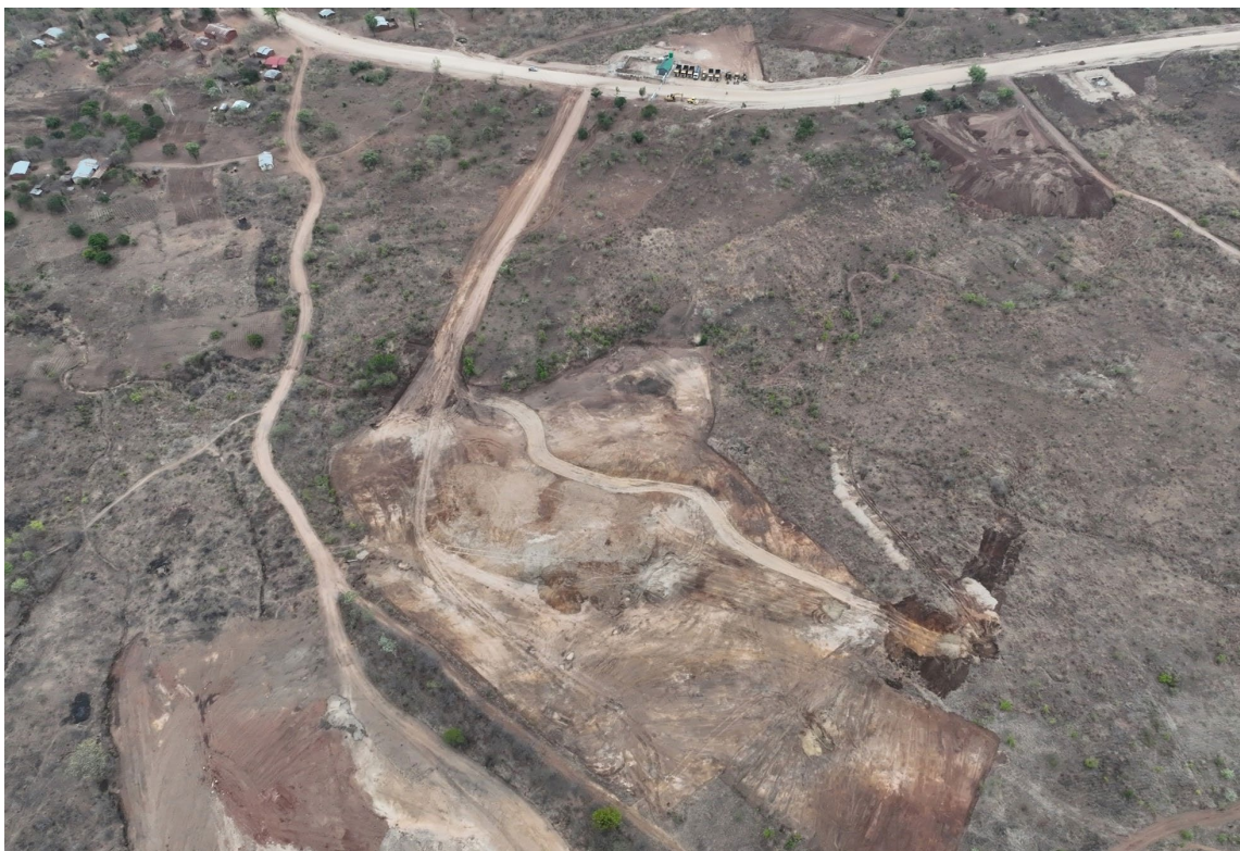
Picture 1. Clearing complete at the future Tipume Camp site at Kangankunde
