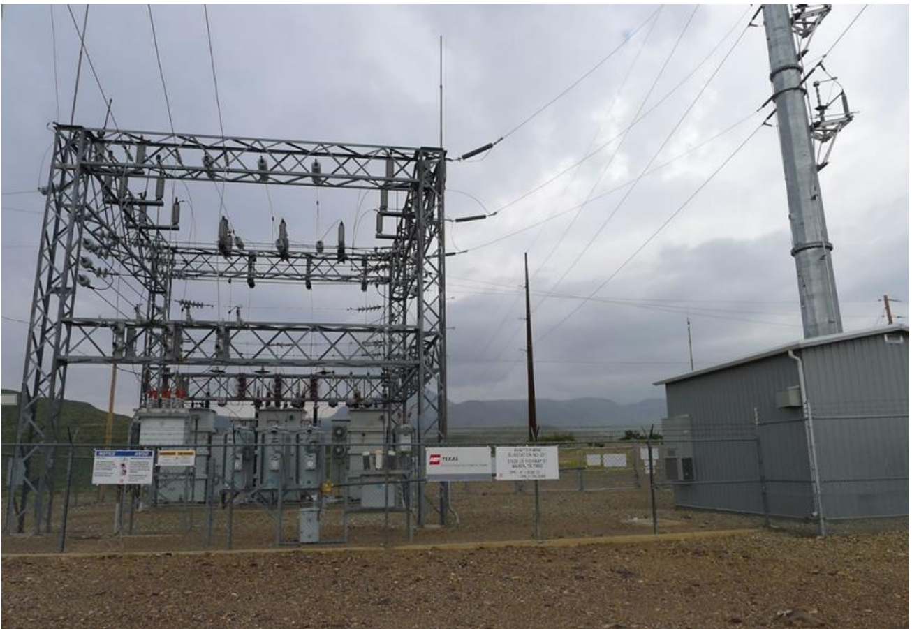
Figure 5: Shafter Mine and Processing Substation.
