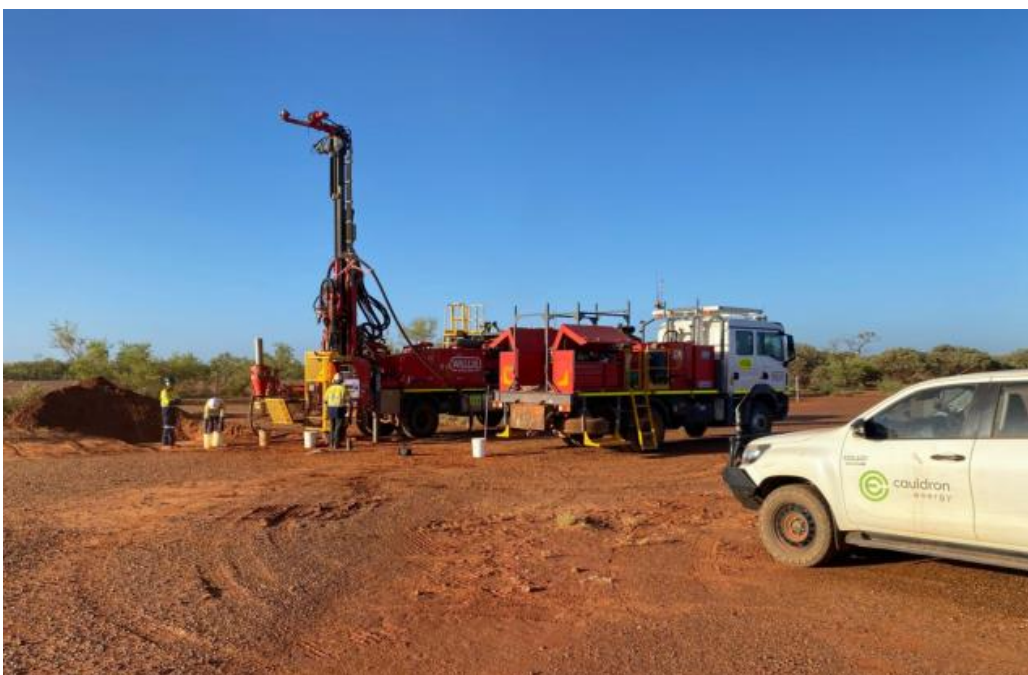
Image 1. Drilling in action at Yanrey.
