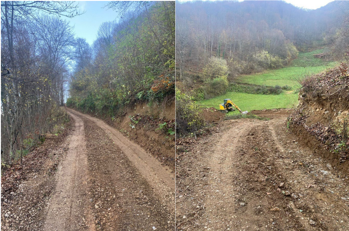
Figure 3: Roads prepared and earthworks completed to access Sinjakovo gold targets.
