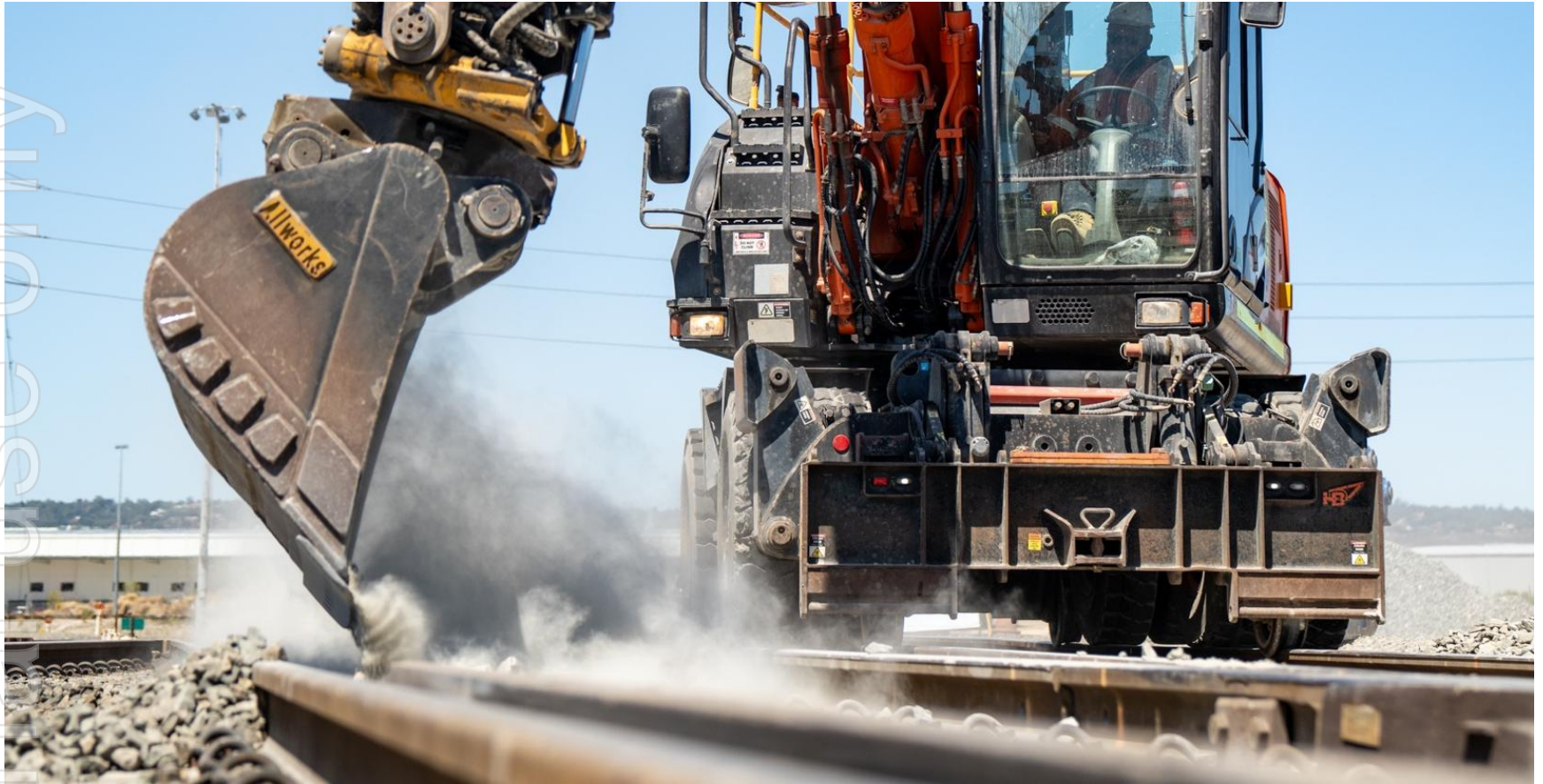
Delivering rail maintenance services at the Perth Freight Terminal, Western Australia.
