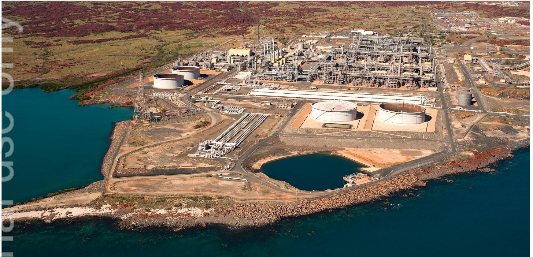
Woodside's Karratha Gas Plant in Western Australia.
