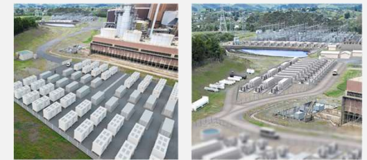
Huntly BESS Stage 1 and 2(1)
