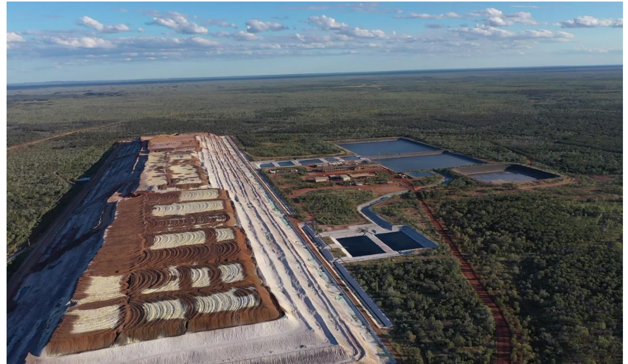
Mount Kelly Copper Processing Facility (Source: Austral Resources)
