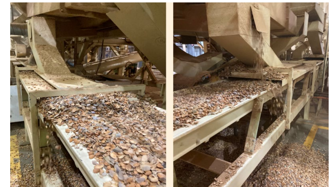
Kernel Conveyance capacity upgrade
