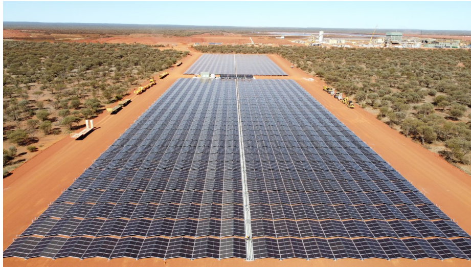
7MW Mt Weld Solar Farm constructed & commissioned 2,376 solar panel sections (with PPA partner Zenith Energy)
