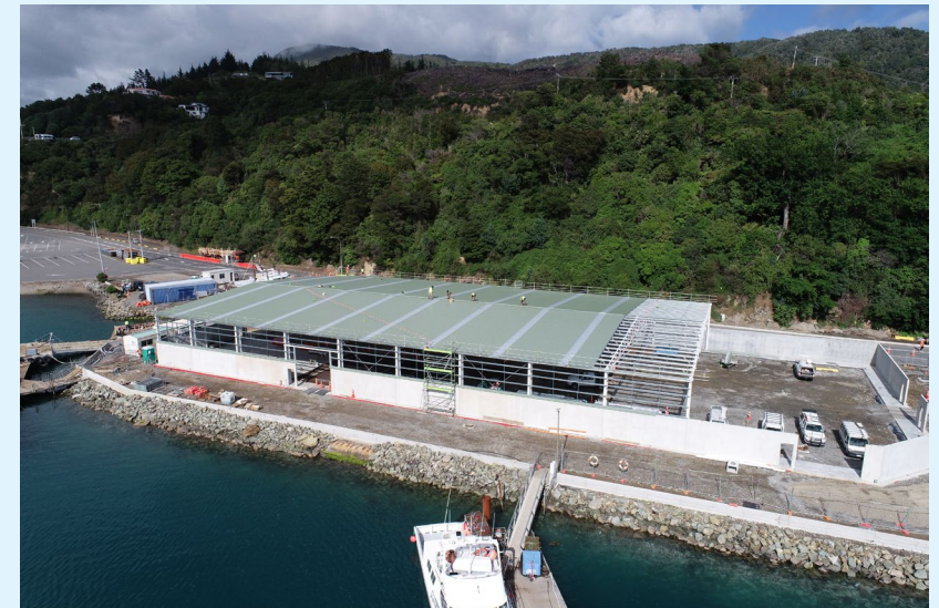
Build of Westshore Warehouse in Picton underway
