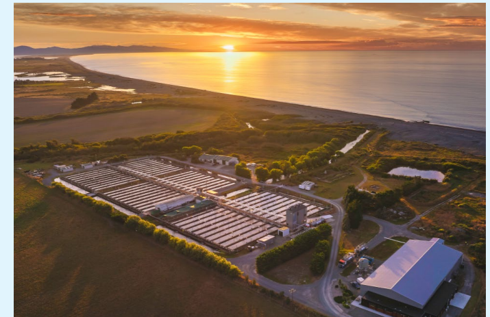
Our Tentburn hatchery facility where our pilot RAS will be located
