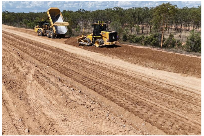
Figure 7b: Earthfill infill placement
