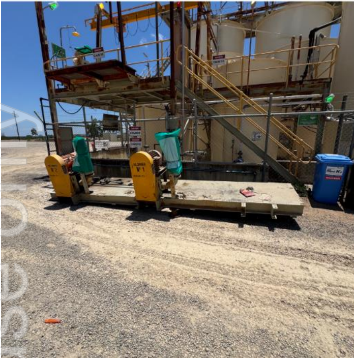
Figure 6e: Removal of previous blower
