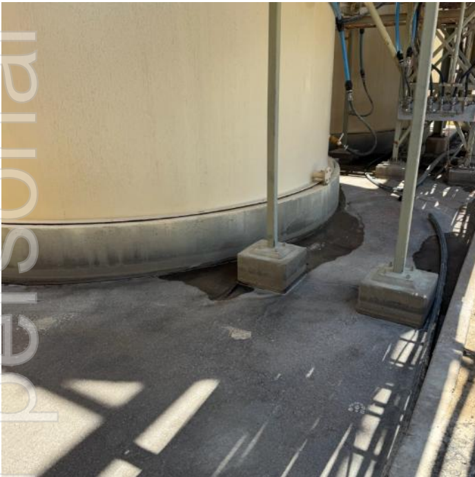
Figure 6g & h: New air sparge system and manifold for the CIL tanks
