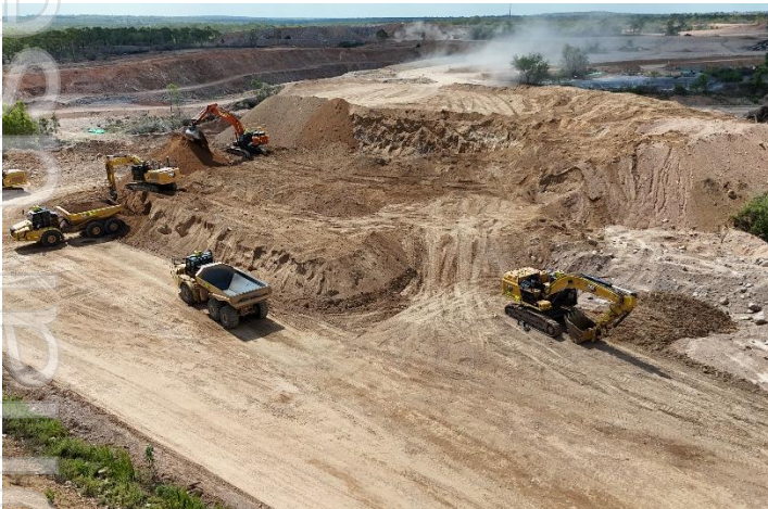
Figure 7a: TSF material stockpile – moisture conditioning
