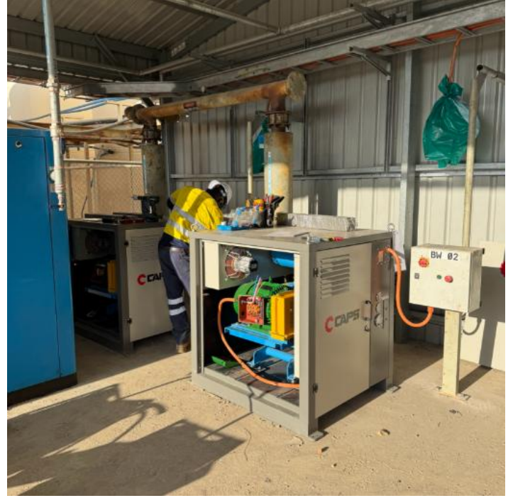
Figure 6f: New blower installation
