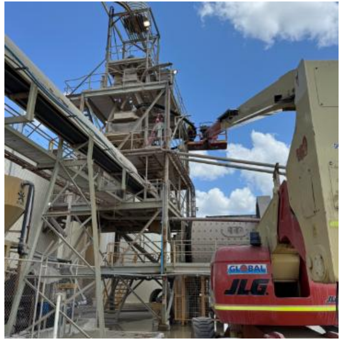
Figure 6b: New mine hose installation
