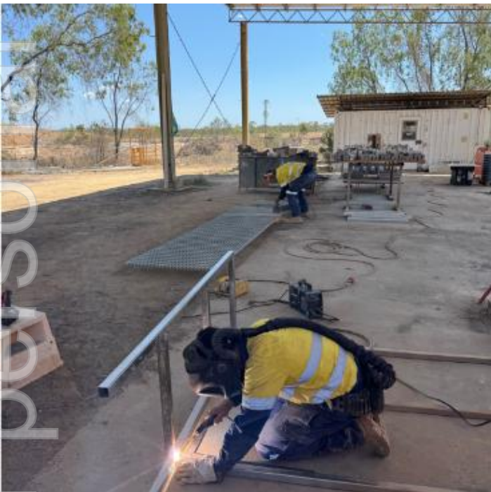
Figure 6c: Ongoing workshop fabrication for overall plant renewal
