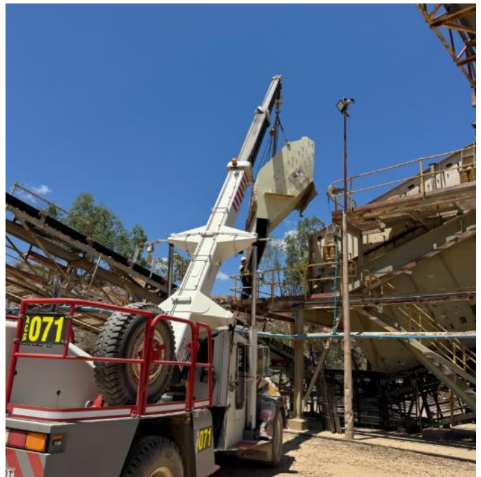
Figure 6d: CV04 chute installation
