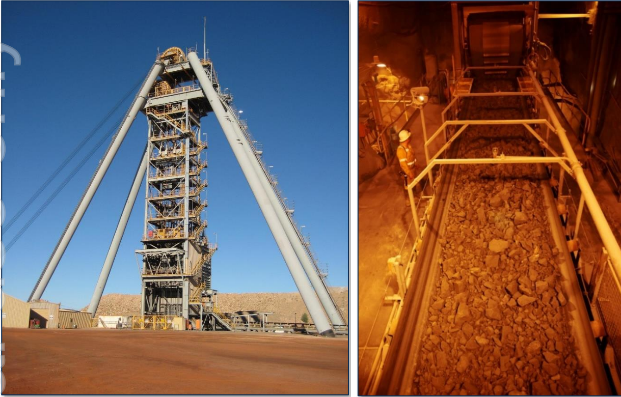
Figure 4: MDU shaft headframe (left), underground conveyor system (right)
