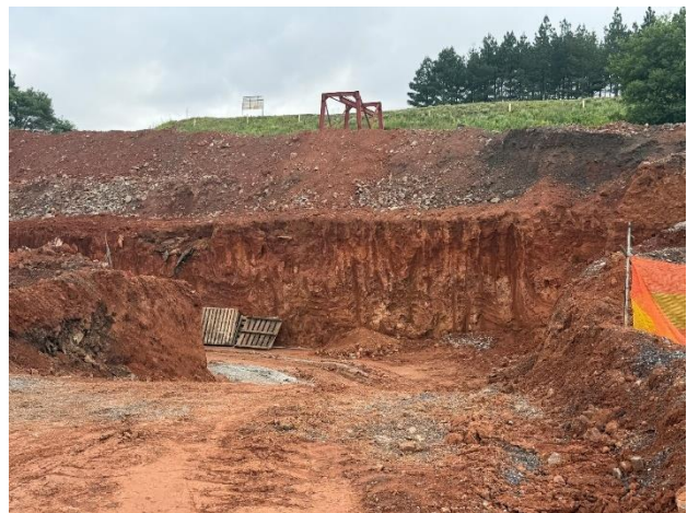
Figure 2: Bulk excavation - concrete retaining walls
