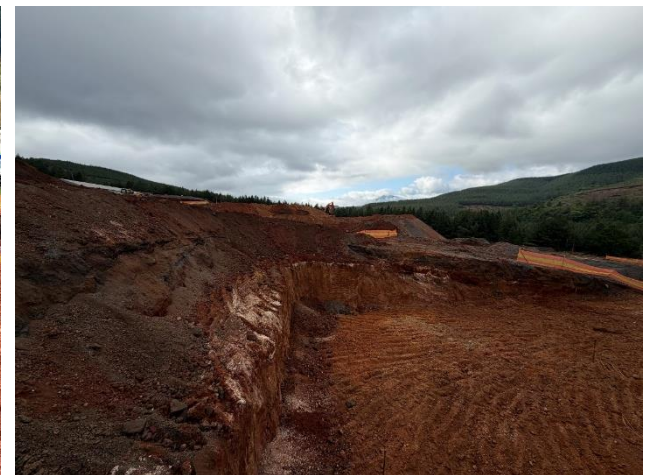
Figure 4: Bulk excavation - gold room platform
