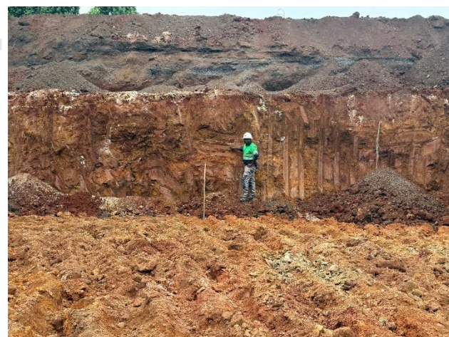
Figure 5: Bulk excavation - gold room platform
