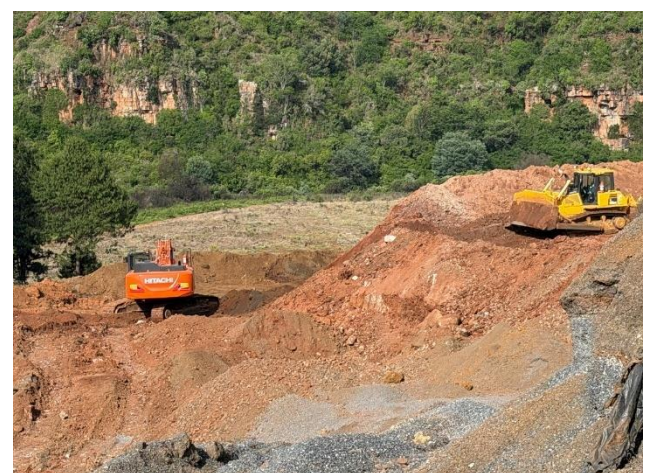
Figure 6: Bulk excavation - platform 3 area
