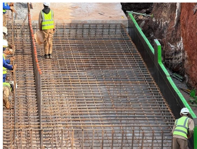
Figure 10: Retaining wall foundation steelworks
