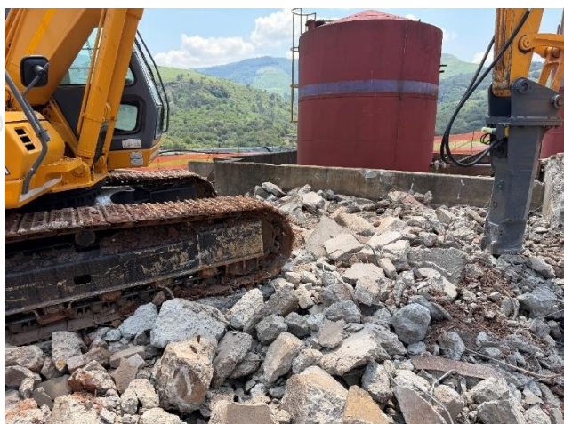
Figure 7: Removing old engineering structures
