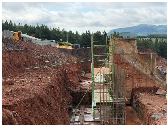
Figure 9: Retaining wall steelworks extensions
