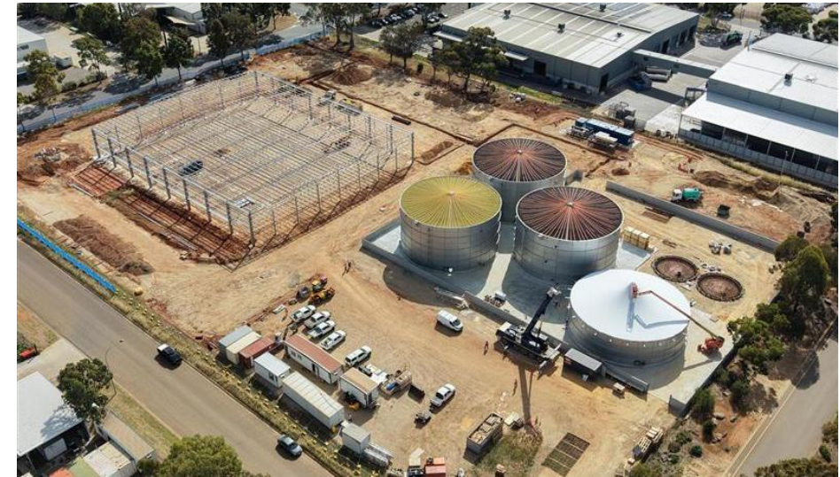
SA1 Salisbury Bioenergy Plant construction, SA
