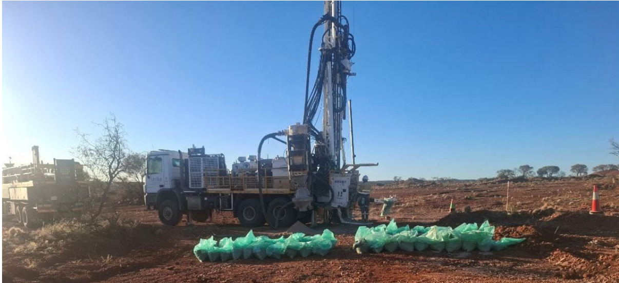
Photo 1: RC Drilling rig on site at Red Dog, Laverton Gold Project
