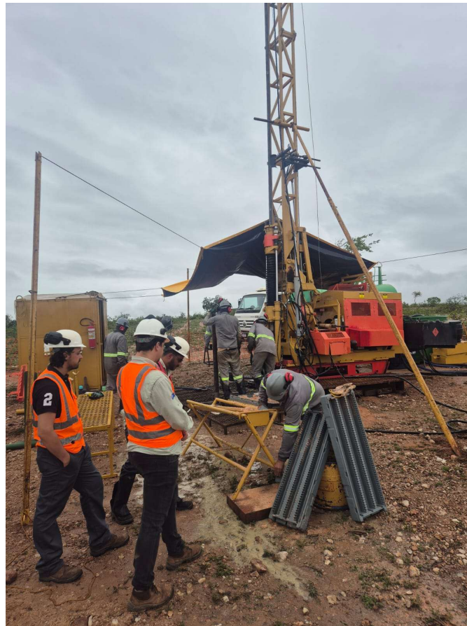
Figure 2: Enova's team closely supervise contractor activities
