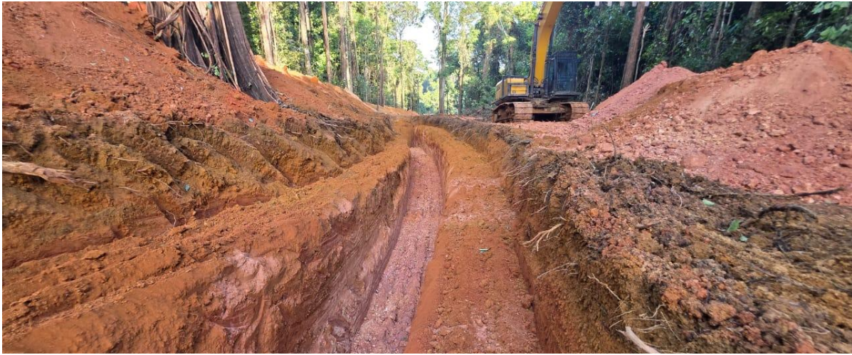
Figure 2: Trench No. 4 at South Oko, looking east, Line 696000N.
