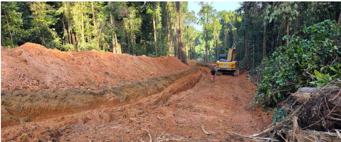
Figure 3: Trench No. 4 at South Oko, looking west, Line 696000N.
