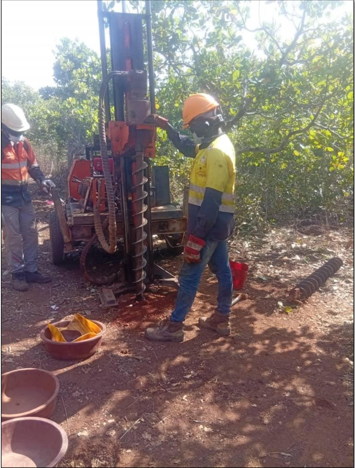
Figure 2: Power auger drilling at Tougbe.
