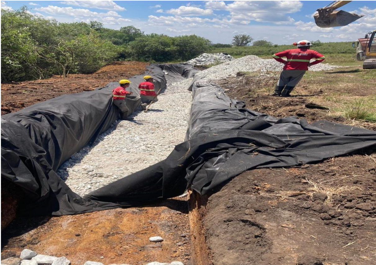
Image 2: Drainage to the sump advancing on schedule.
