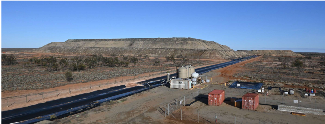
Photo 2: SART plant (foreground) and heap leach pad (background)
