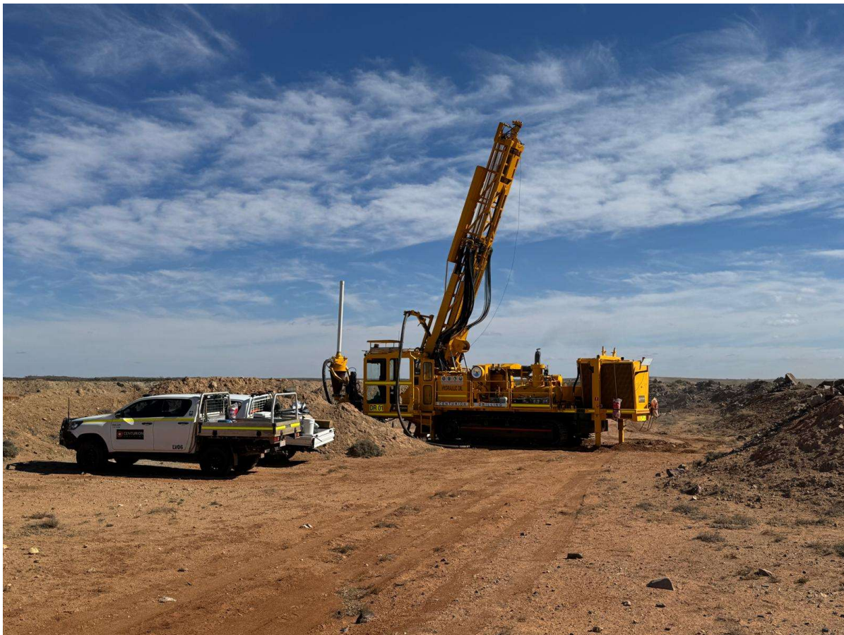
Photo 2: Vertigo RC Drilling underway at the White Dam Gold Project, South Australia.
