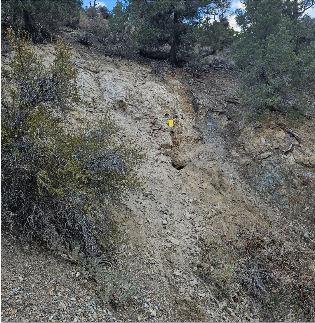
Figure 1: Collapsed historical adit on a 4m wide faulted zone at Dollar project, Nevada.
