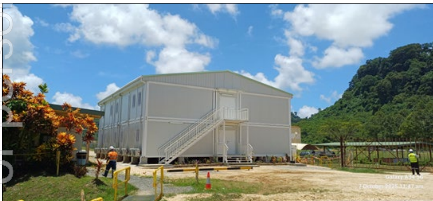
Figure 4: New Environment and Mine Technical Services Office
