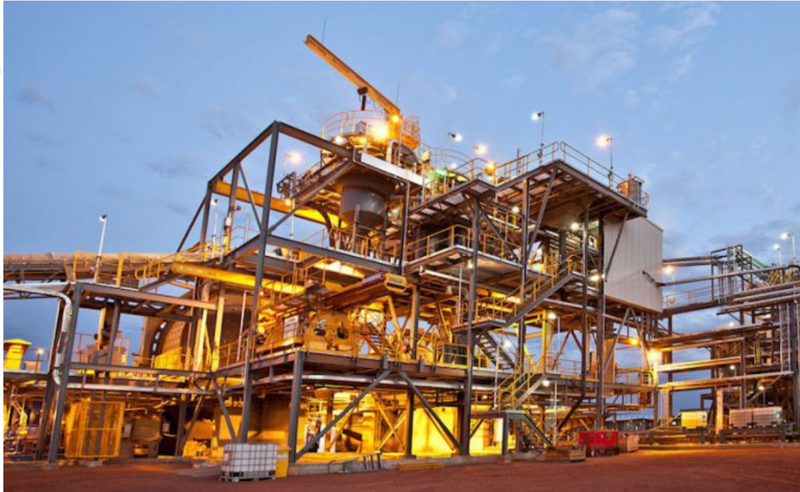
Figure: The DeGrussa Processing Plant
