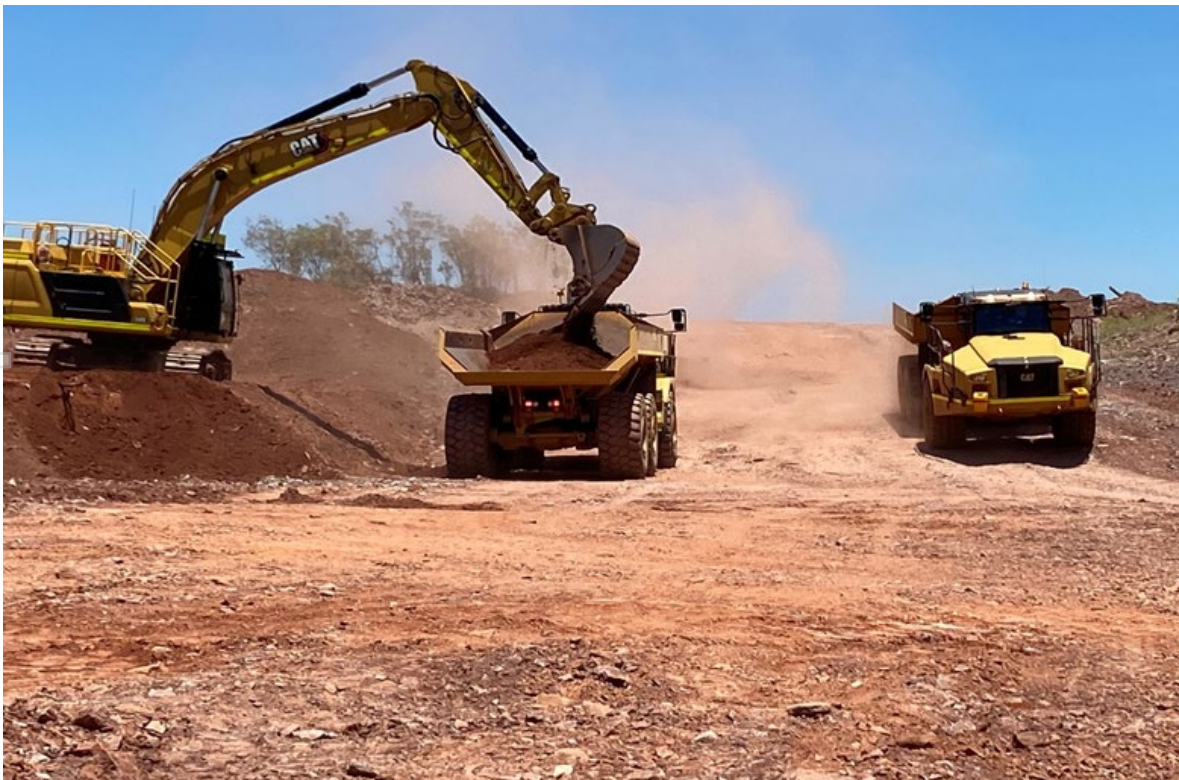
Figure: Early Works Excavation
