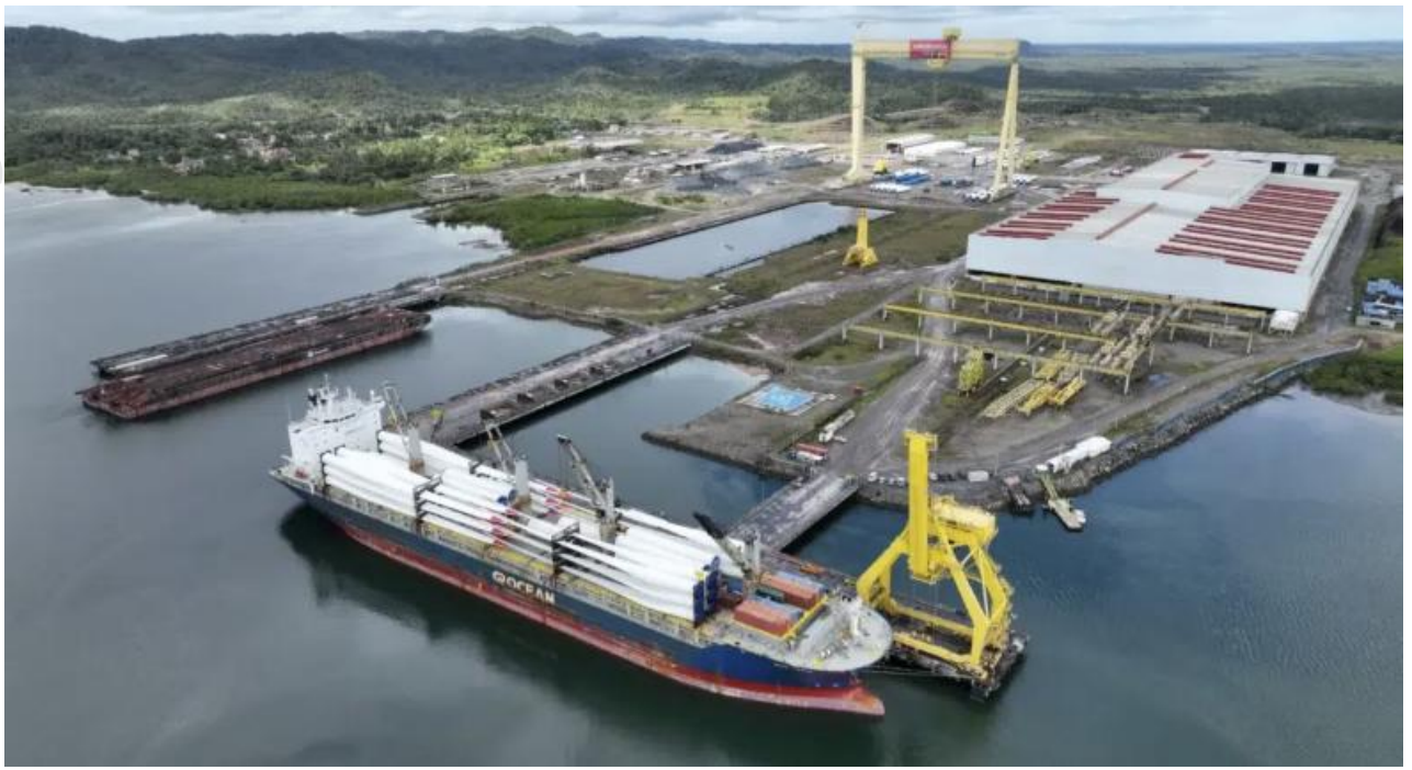
Figure 22: Port of Enseada – Deepwater Export Facility
