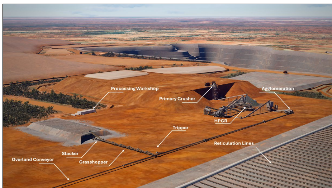
Plate 2 – Apollo Hill Gold Project PFS Design rendered visualisation – Conceptual stacking of crushed ore onto Phase 3 Heap Leach Pad. Foreground shows reticulated pipework for delivering leach solution to drippers for percolation of leaching fluid through heap leach pad. Apollo Hill PFS pit design in background and crushing circuit and ROM pad in middle field of view.
