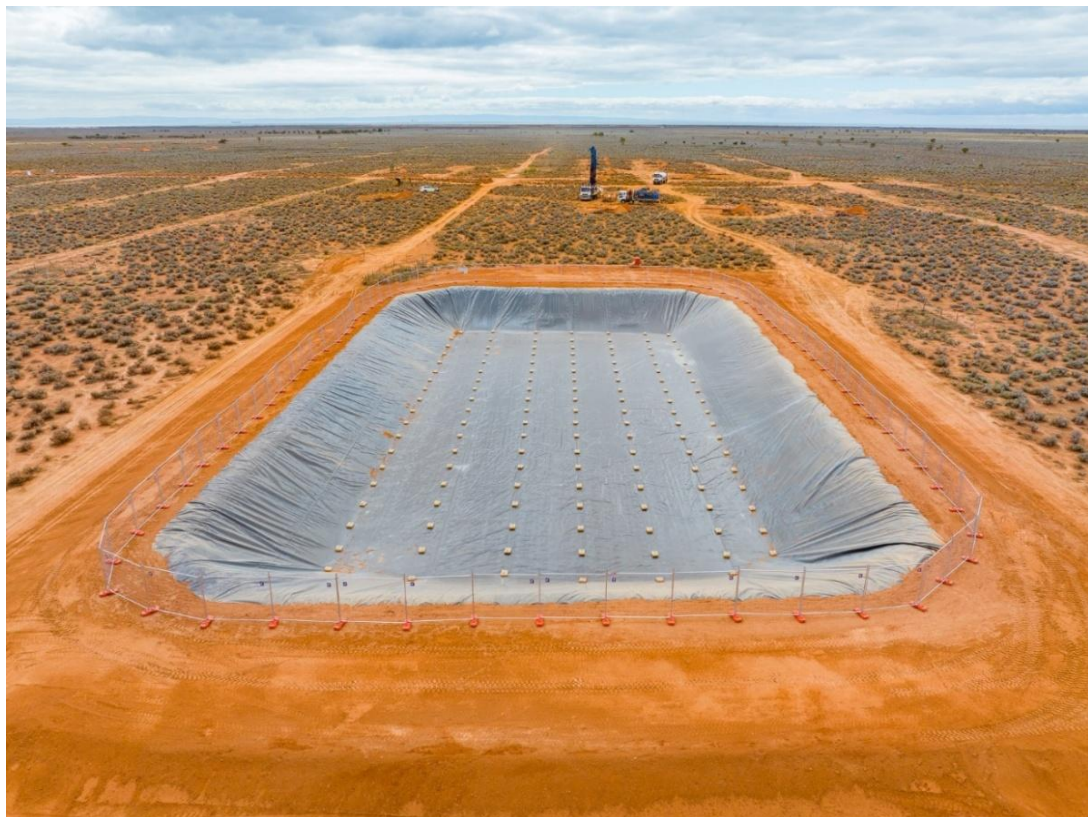
Figure 5: Lined Pond Used For Hydrogeological Testwork Associated With The Trial
