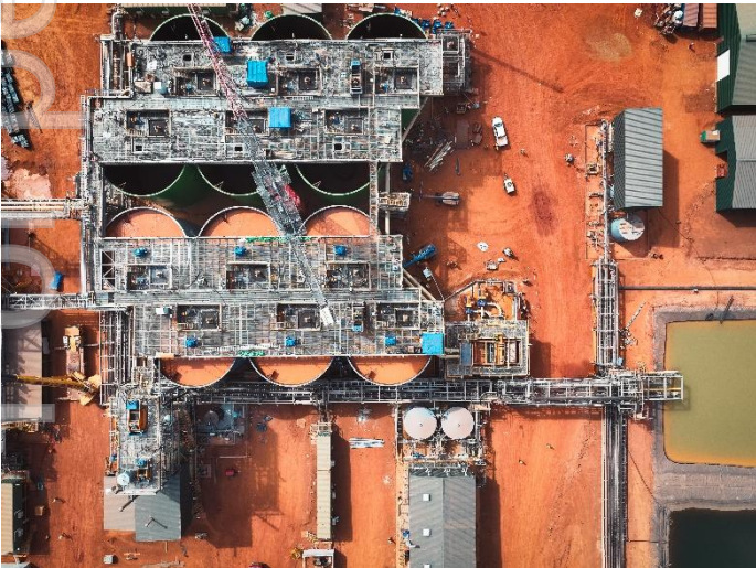
Figure 7: Train A CIL Tanks Gold Processing
