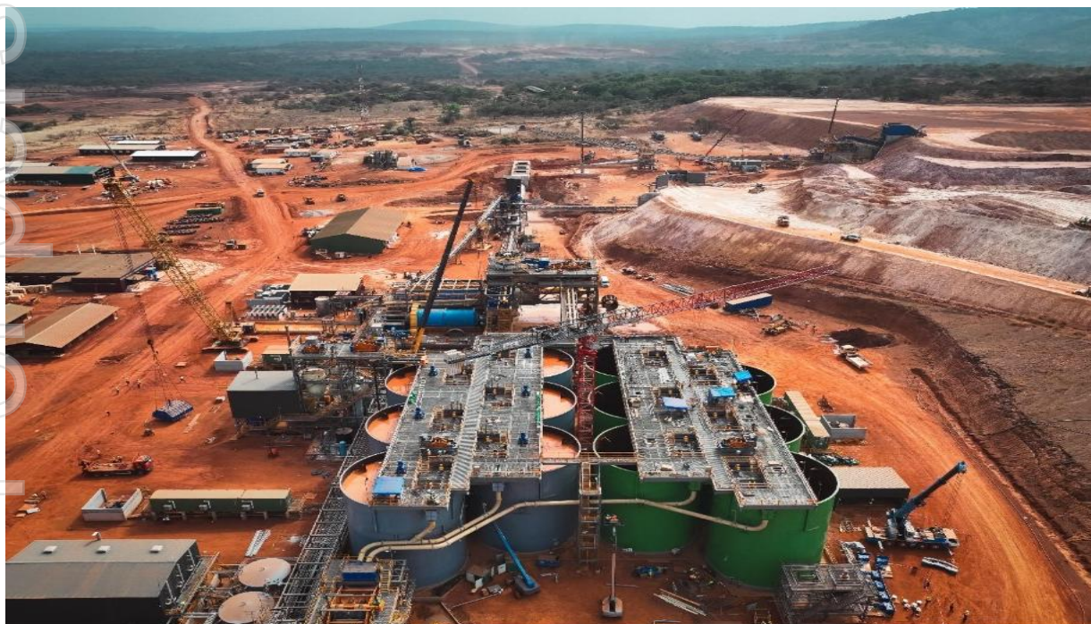
Figure 2: Aerial View of the Kiniéro Gold Project – Ore Delivered to Train A CIL Tanks
