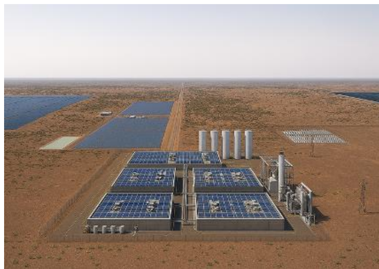
Figure 2: Aurora Continuous Energy Hub concept - impression of data centre with 1414 Degrees TESS, solar PV and BESS, connected to the NEM via the 275kV transmission line powering mines to the north of the Aurora Precinct.
