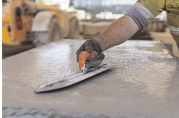
Figure 3 & 4: Wind farm concrete trials - 50% AusPozz™ mix design
