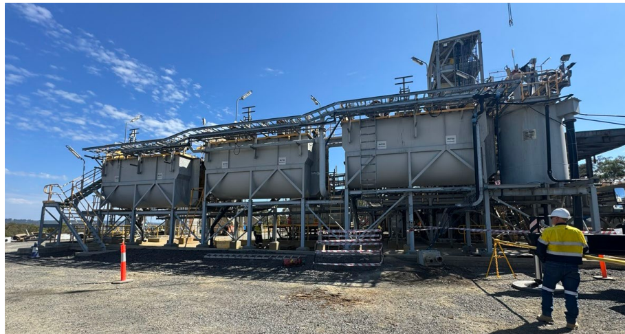
Figure 1 Removal of services from the Flotation Area
