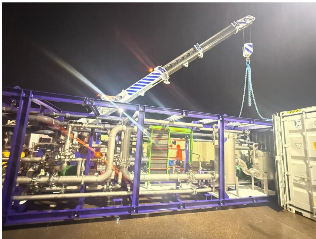
Figure 2. Load out of nano-filtration plant
