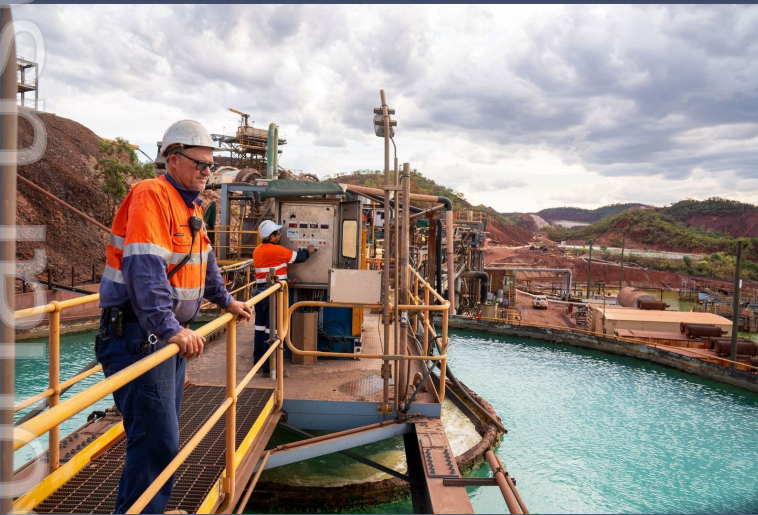
Processing plant & surface infrastructure
