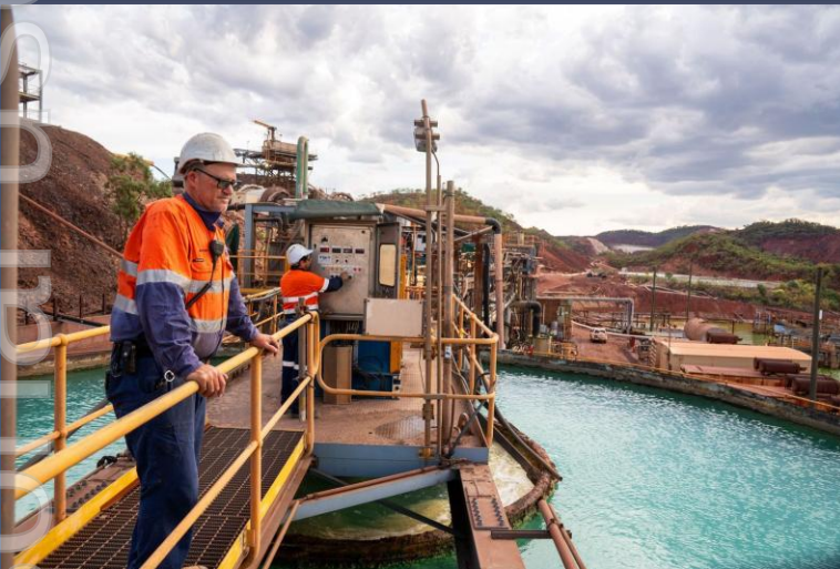
Processing plant & surface infrastructure
