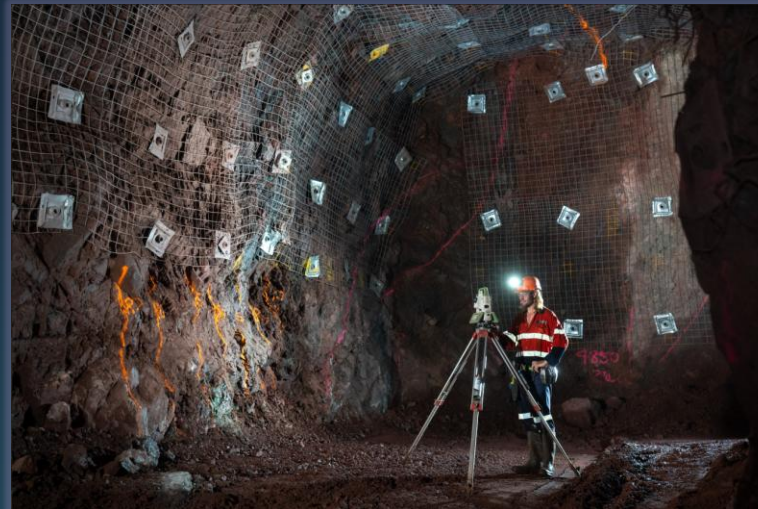
Established underground development
