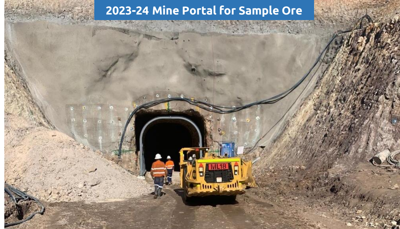
Demonstration Plant Concentrator
