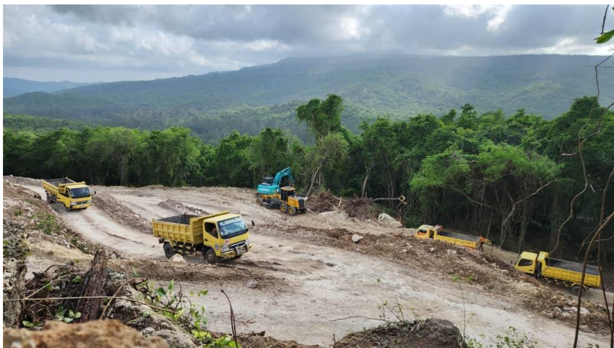
Figure 2: excavation teams mobilised to Ira Miri.
