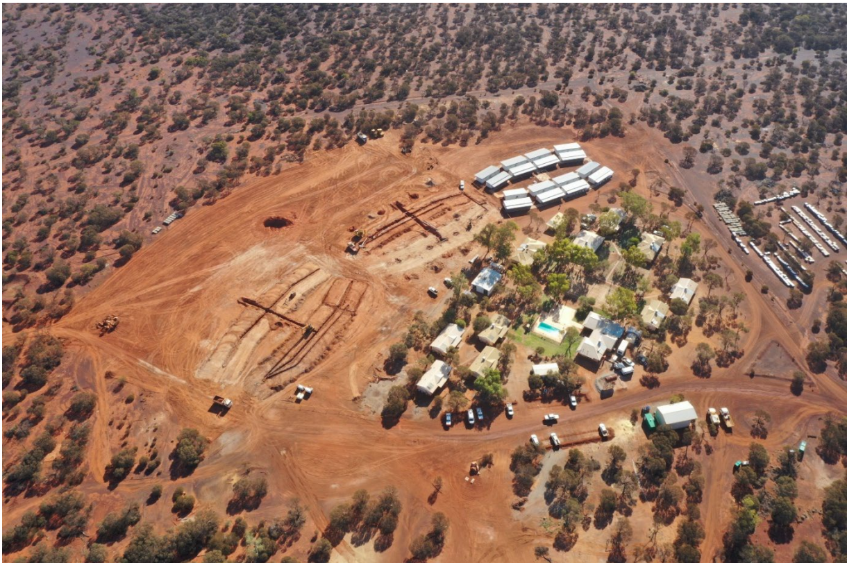
Figure 5 – Camp and expansion works
