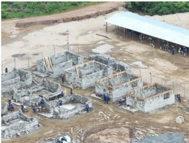
Pictures 5 & 6. Progress at the site camp facilities, showing completed foundation excavations, construction of VIP accommodation units, and advancement of Mess Hall, BQ accommodation and entrance earthworks supporting upcoming project mobilisation
