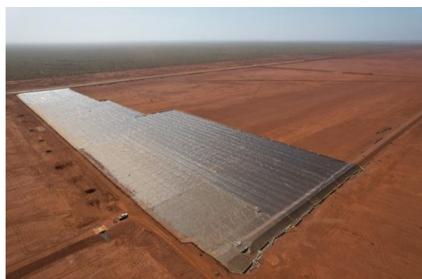
Figure 4: Crystalliser pond lining
