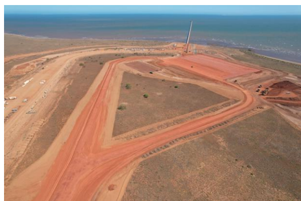
Figure 6: Stockyard earthworks
