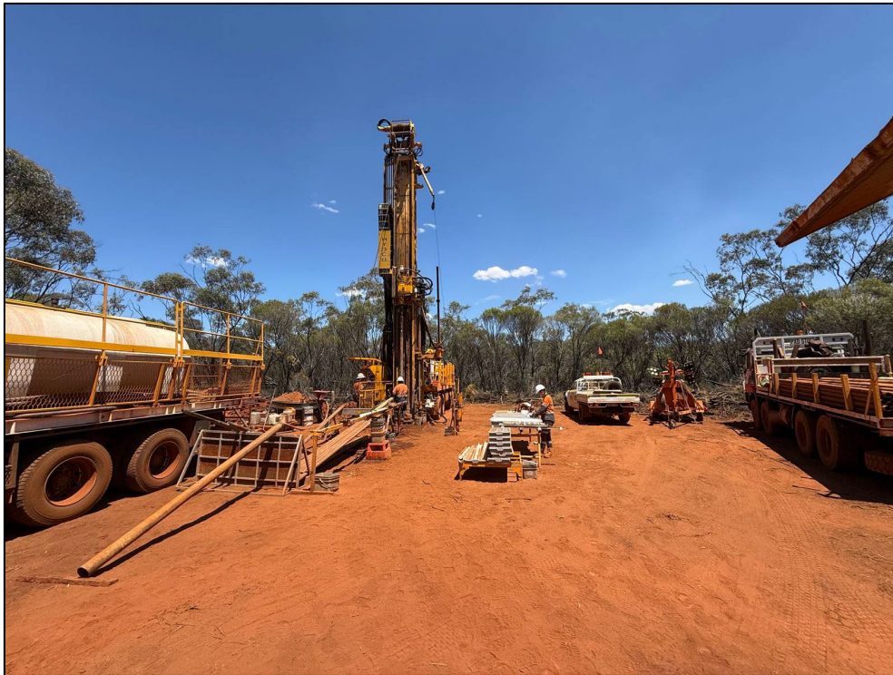
Figure 7 – Diamond drilling to support the tailings storage facility design
